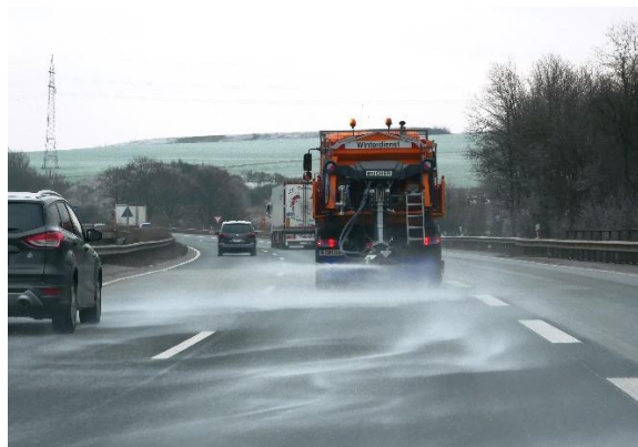
Figures 22 and 23: Application of 15 g/m 2 salt (fine grained) with a spreading width of 6 m at 50 km/h, left: prewetted salt FS30, right: dry salt.
